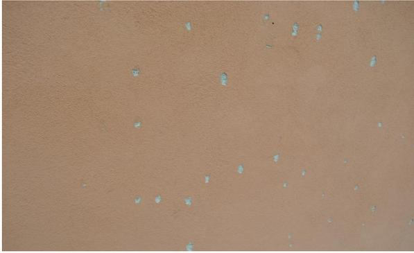
**Fig. 4.** Low resilience of current used retrofit methods – hailstone impact points
