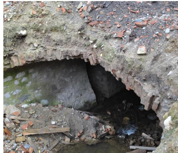
**Fig. 11.** Collapse of a part of the existing vault
