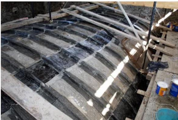
**Fig. 13.** Positioning of FRP: bi-directional strips (<http://resimix.com/categorie-di-intervento/rinforzo-volte> - 02/05/16).
