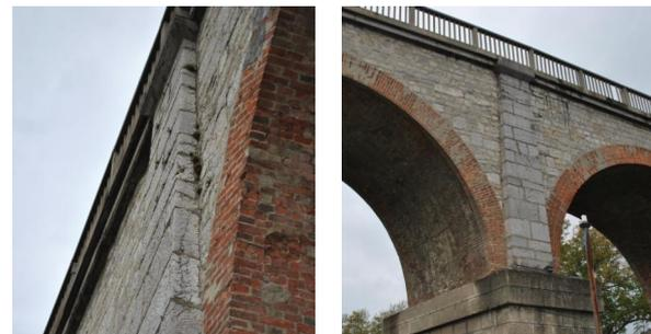
**Fig. 14.** The viaduct from Oravita - different state of conservation of the two faces
