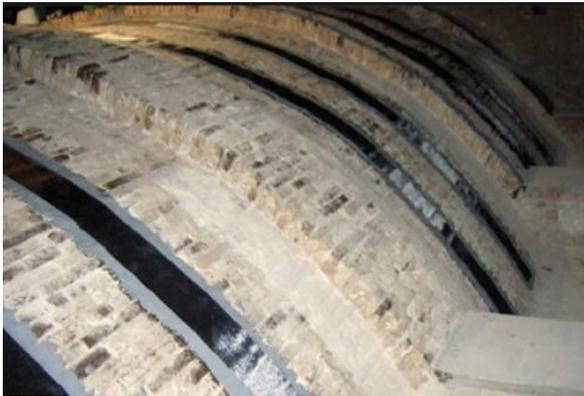
**Fig. 12.** Positioning of FRP: unidirectional strips (<http://resimix.com/categorie-di-intervento/rinforzo-volte> - 02/05/16)
