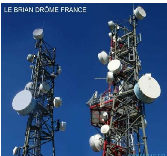
Fig. 2. Hertzian Parabolic Repeaters of mobile phones systems: deterioration and impact over the environment - overhead view (Next-up organisation France, 2012)
