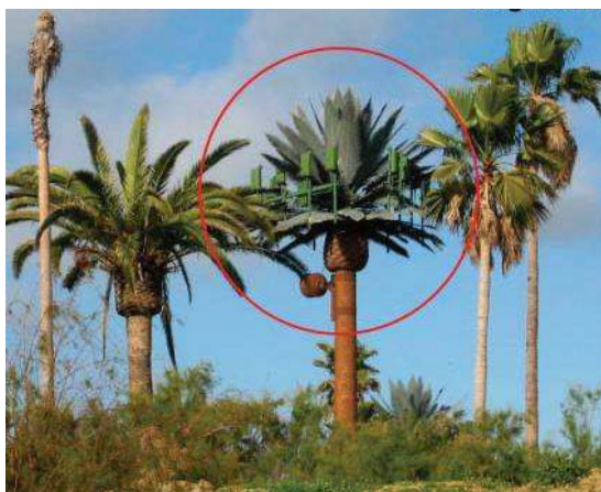
Fig. 3. Cell towers disguised as trees (Rees and Havas, 2009)
