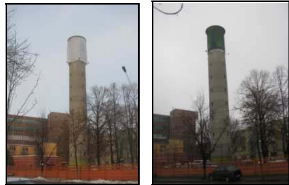
Fig. 2. The water tower in the Pantelimon (Bucharest) borough before and after painting
