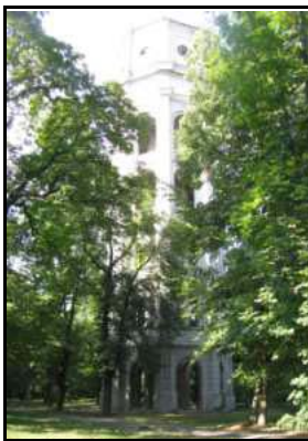
Fig. 4. The water tower in Buftea
