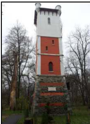
Fig. 11. The Water tower in Târgu Jiu
