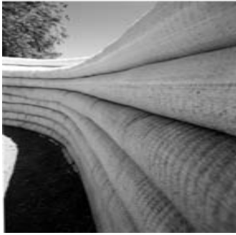
Fig. 1. Wall of Superadobe construction
