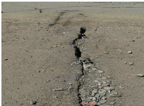
Fig. 1. The settlement of county road, cracks in the asphalt pavement
