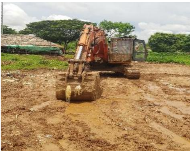
Fig. 4. Lake Neutral site, Bhubaneswar, India - dredging in progress (Source: Authors).
