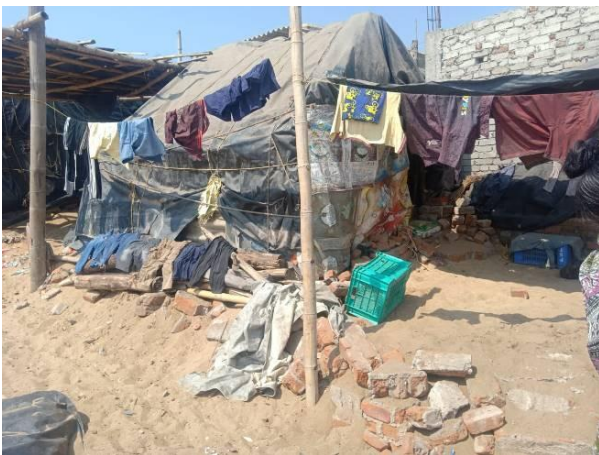
Fig. 11. Cyclone affected the houses of Penthakata (Source: Authors).
