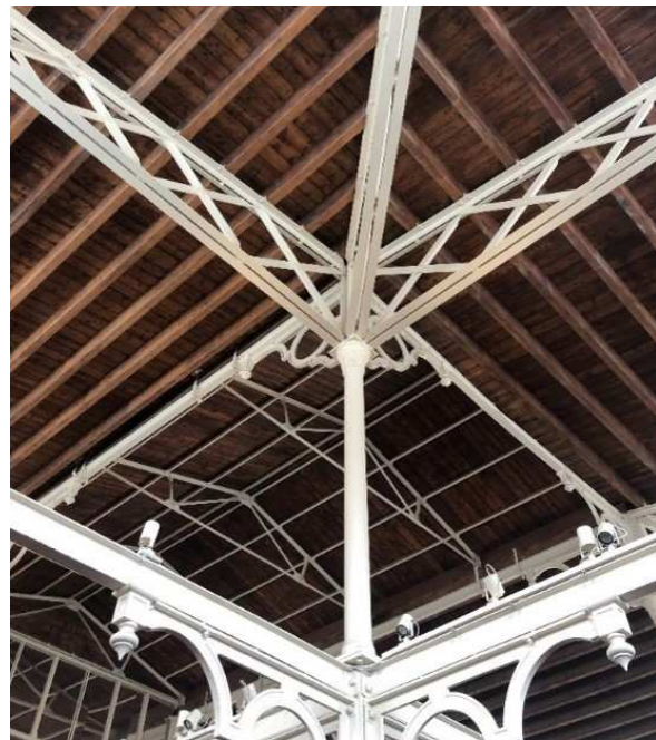
Fig. 17. Reconstructed timber roof.
