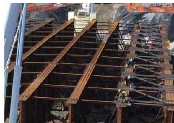
Fig. 10. State of the girders before and after repair ( https://www.cbc.ca/news/canada/edmonton/groat-road-bridge-twister-bender-or-bucky-edmontonians-suggest-names-1.3079412 ).
