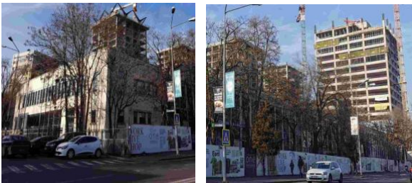
Fig. 10. Ford Branch Assembly: a) administrative building b) industrial hall (Merciu C., January 2020).
