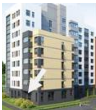
Fig. 4. The designed color scheme of the facades of a residential building with the painted place being indicated.
