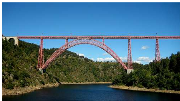
Fig. 3. Garabit Viaduct is a historic monument since 1965.
