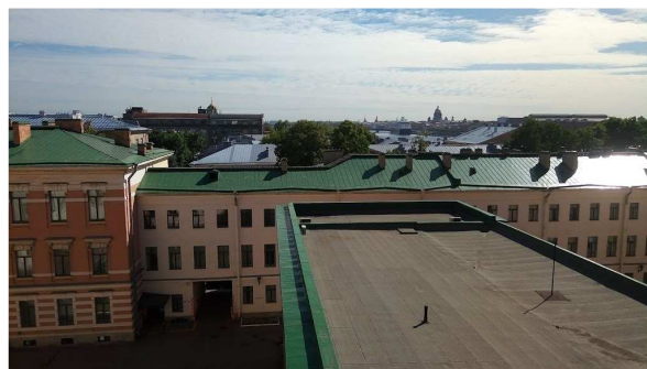
Fig. 3. Roofs of historical buildings of St. Petersburg. The view on St. Isaac's Cathedral.
