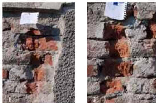
**Fig. 3.** The placement of explosive devices and the effects after detonations
